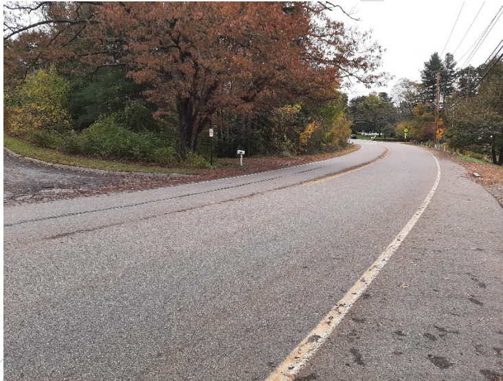
Figure 14: Poor Sightline from Jenkins Drive as Bartlett Curves
