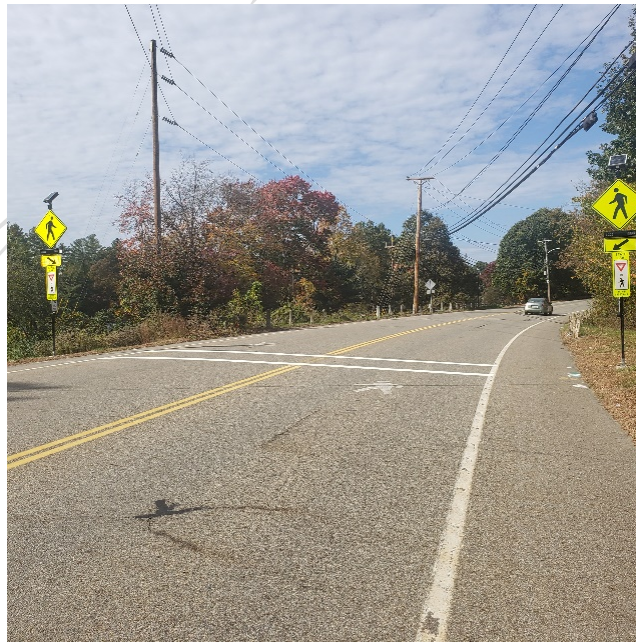
Figure 18: Bartlett Street Crosswalk with RRFB Signal
