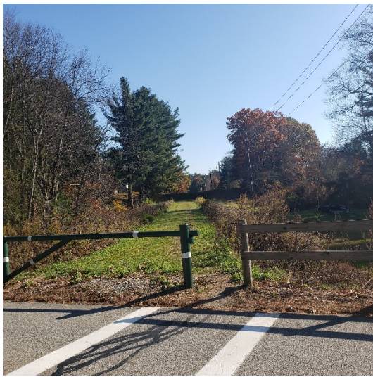
Figure 10: Aqueduct Trail on Maple Street
