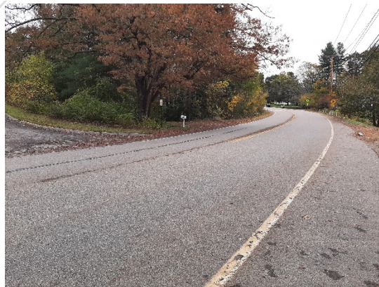
Figure 44: Brush Impedes Line of Sight
