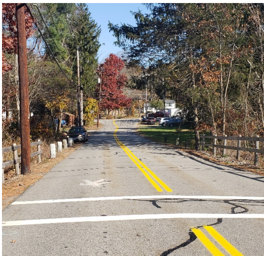
Figure 11: Crosswalk on Maple Street
