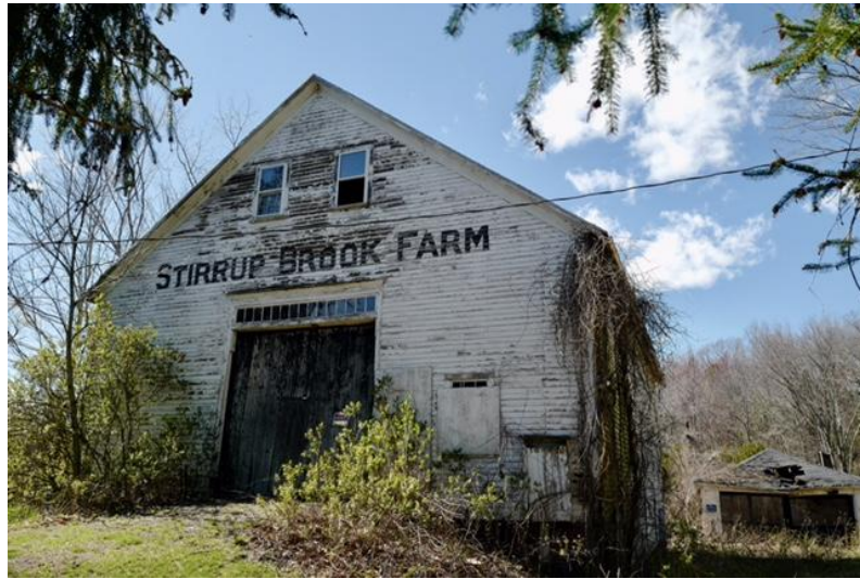
Figure CS-9 Stirrup Brook Farm Barn in 2022 (Photo Courtesy Susan Licht)
