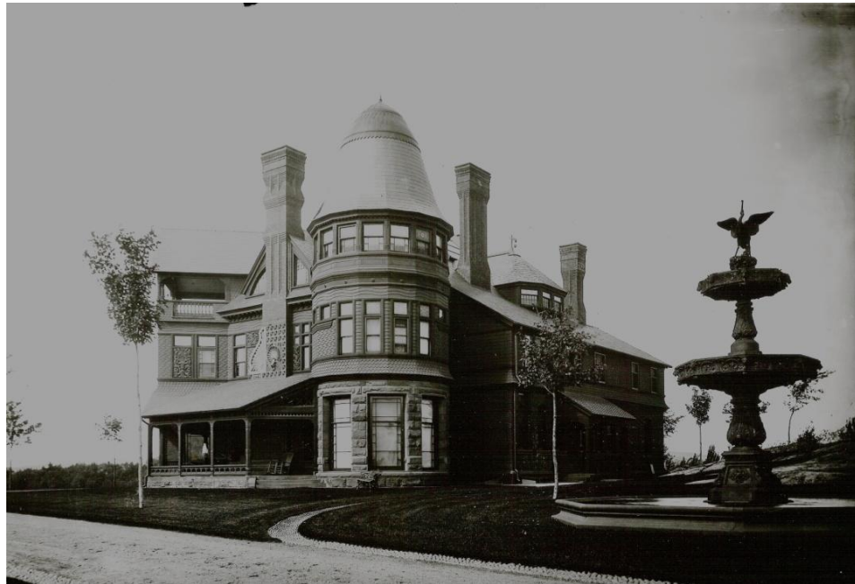
Figure CS-3 White Cliffs Mansion, shortly after construction, circa 1886 (Photo courtesy of the Northborough Historical Society)
