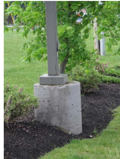
Incorrectly installed light post
